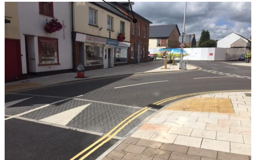
Side road entry treatment and carriageway reduction (Tiverton)
