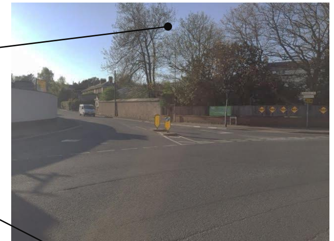
Problematic junction (item 2)
