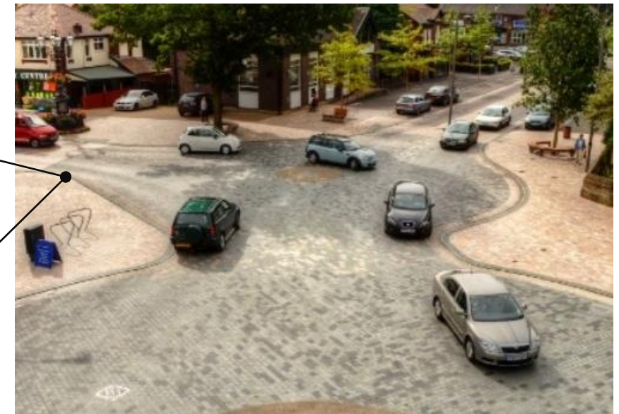
Example of roundel junction (Poynton)
