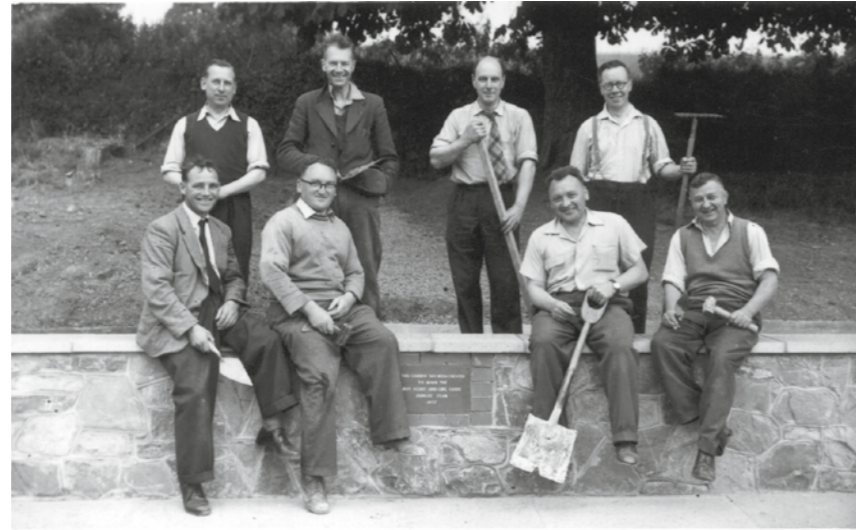
The team of builders, 1957
