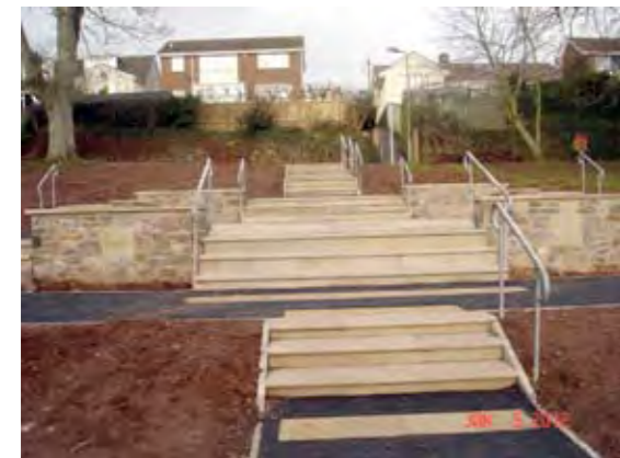
The project in progress, January 2012
