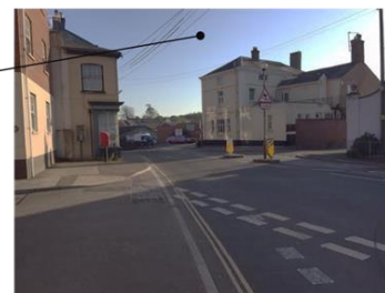
Problematic junction (issue 4)
