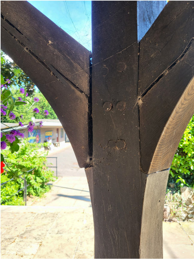
Image 5: Cracks to uprights. No change.
