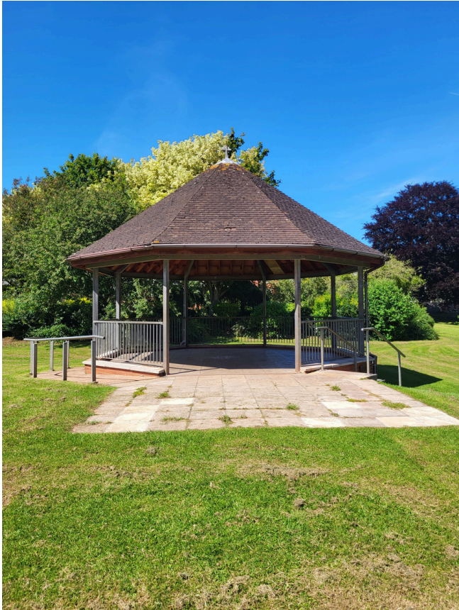
Image 1: Two missing roof tiles at the front
