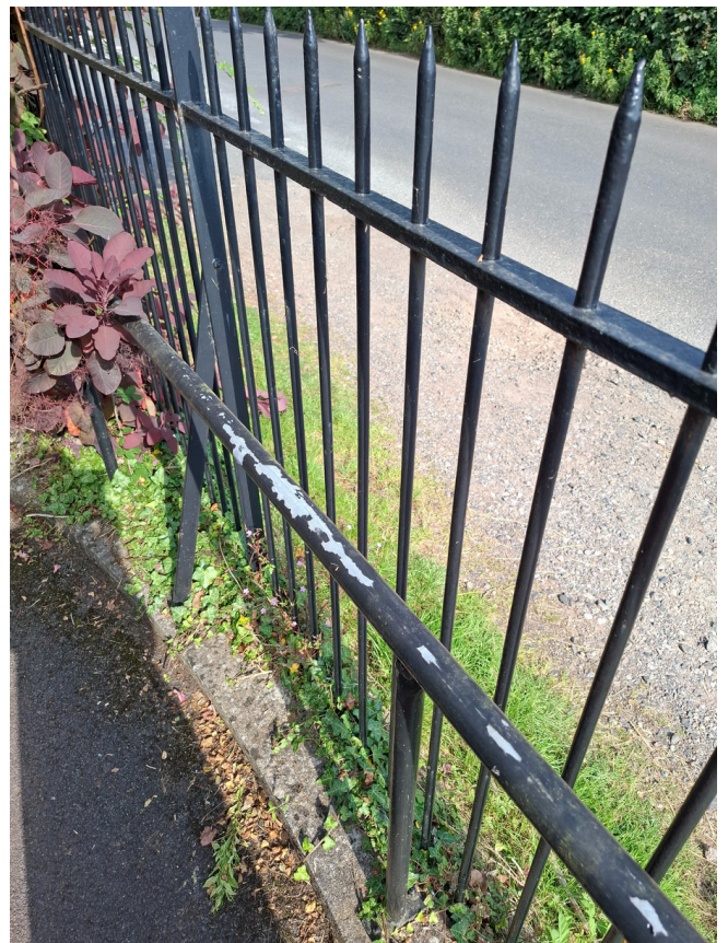
Image 4: Painting peeling on internal handrail
