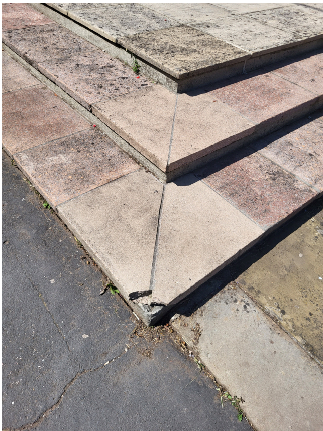
Image 7: Corner of slabs broken
