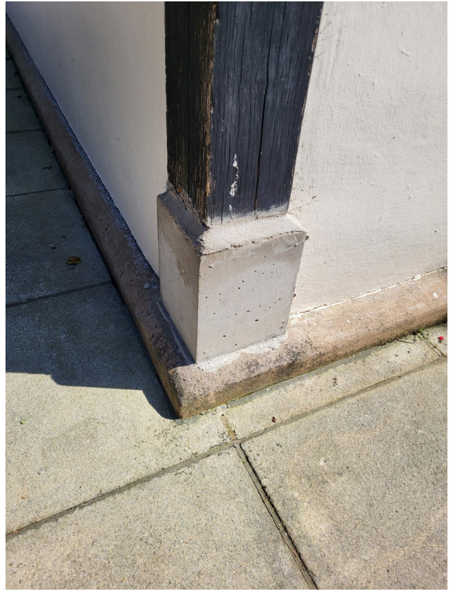
Image 10: Corner plinth rebuilt in November 2023
