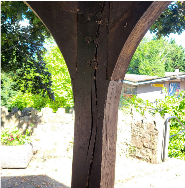
Image 6: Cracks to uprights. No change.
