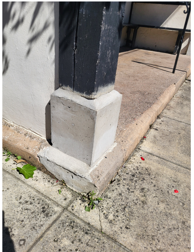
Image 12: Corner plinth rebuilt in November 2023
