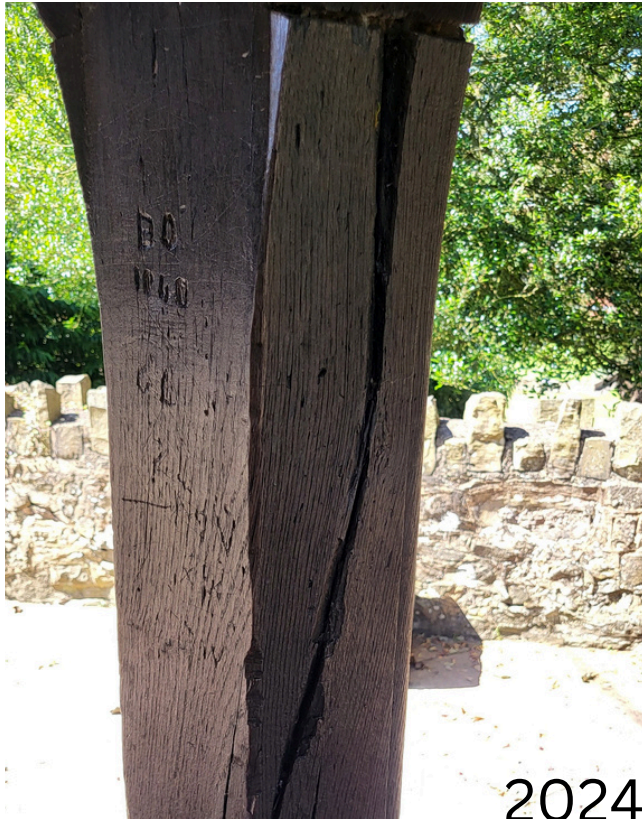
Image 7: Cracks to uprights. Comparison of 2023 and 2024.
