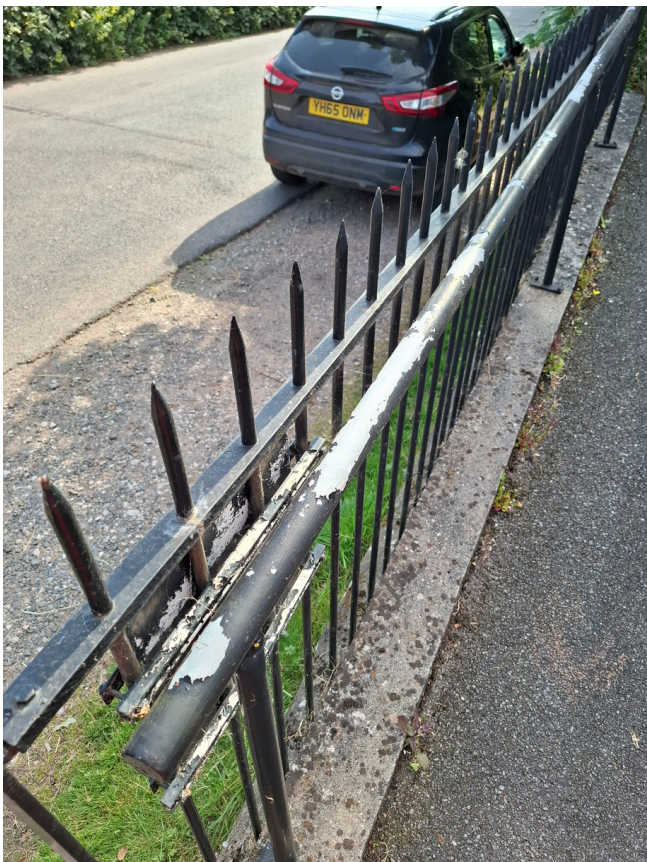
Image 3: Painting peeling on internal handrail
