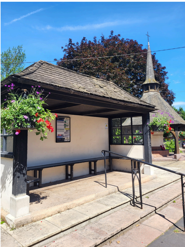
Image 8: Missing and warped roof tiles. No change from 2023
