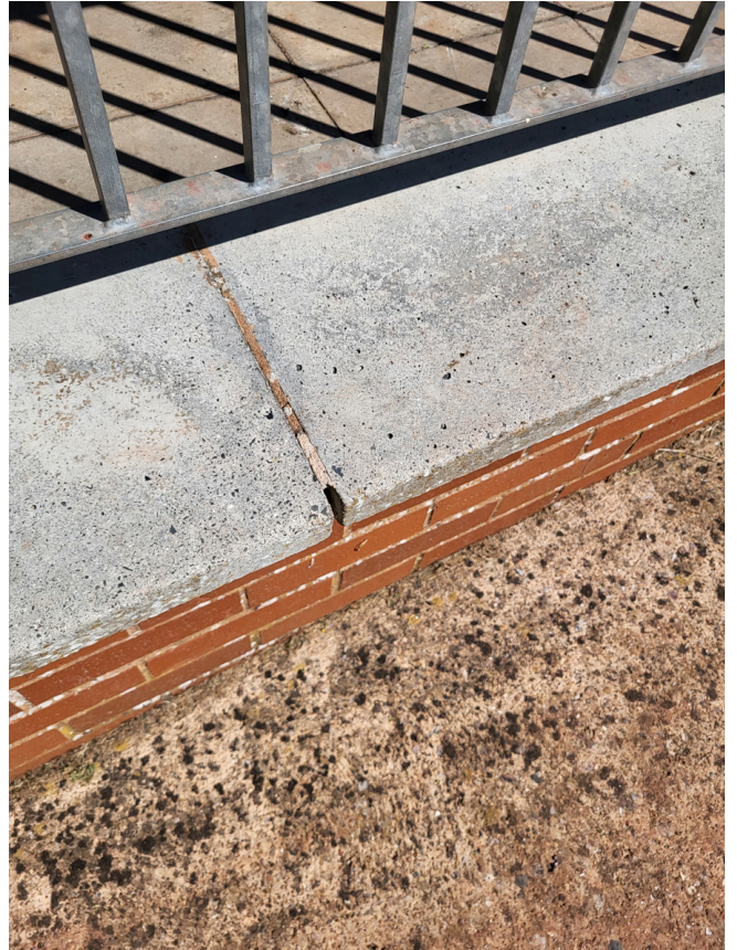
Image 10: Small section of pointing missing
