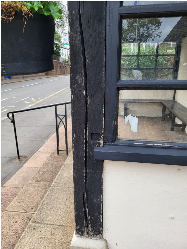
Image 10: No change in cracks to uprights
