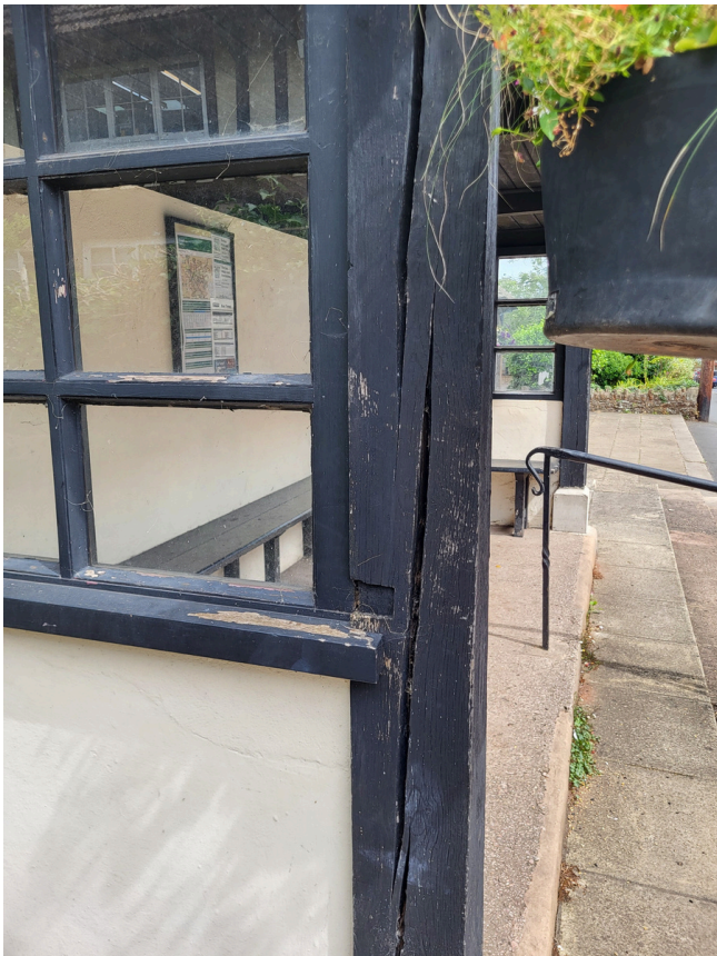
Image 8: No change in cracks to uprights
