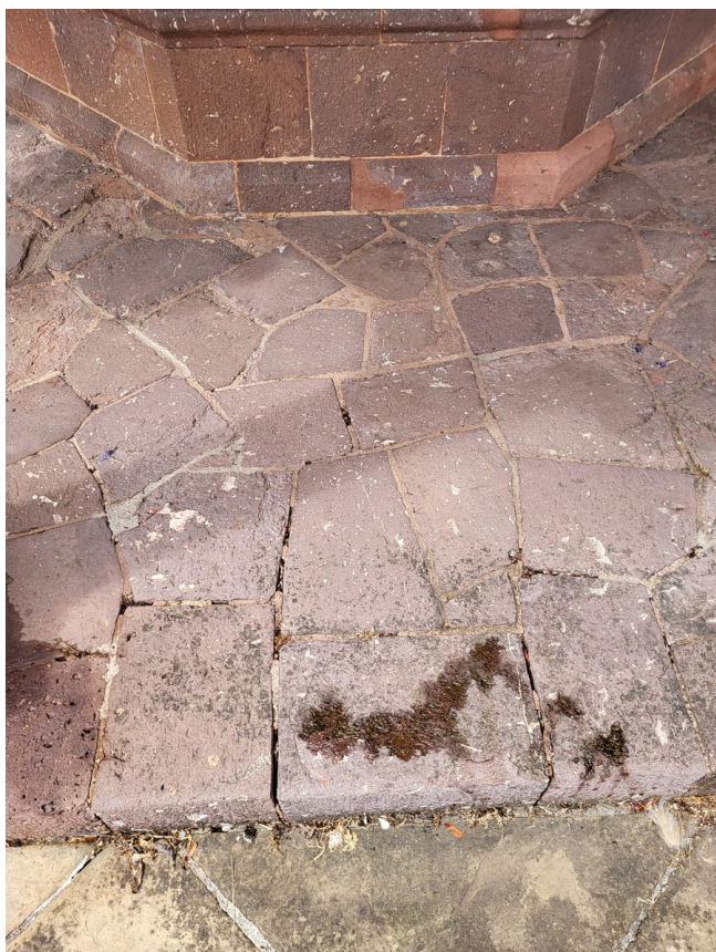
Image 3: Sections of internal slabs need repointing
