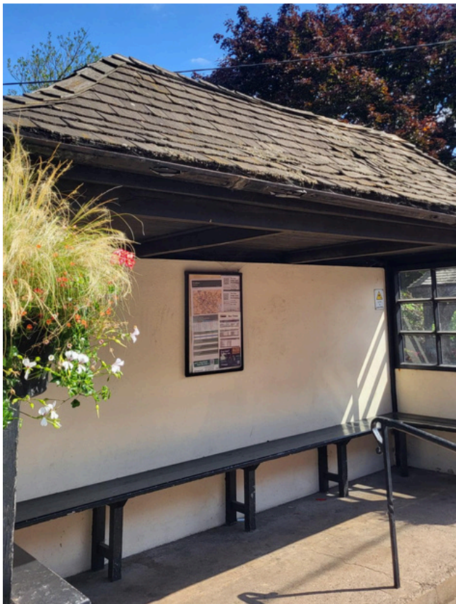
Image 7: Missing and warped roof tiles. No change from 2023/2024
