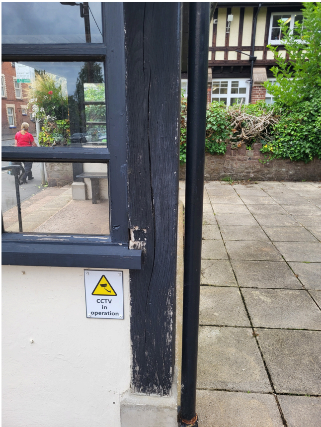
Image 11: No change in cracks to uprights
