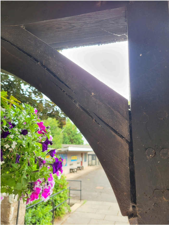
Image 5: Cracks to uprights. No change.
