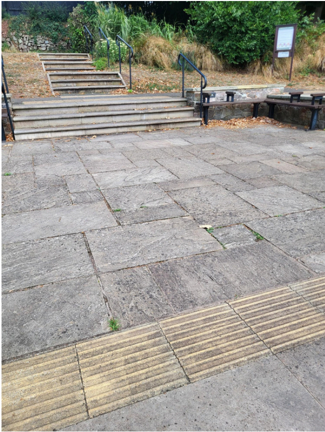
Image 5: General movement and rocking to central slabbed area
