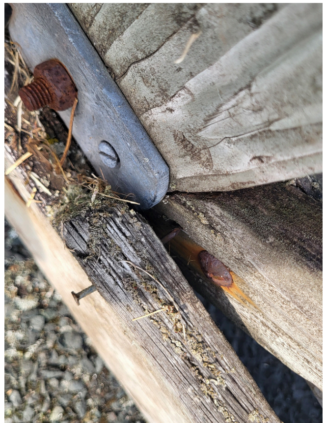
Image 4: Exposed nail and loose wood on bottom rail of gate
