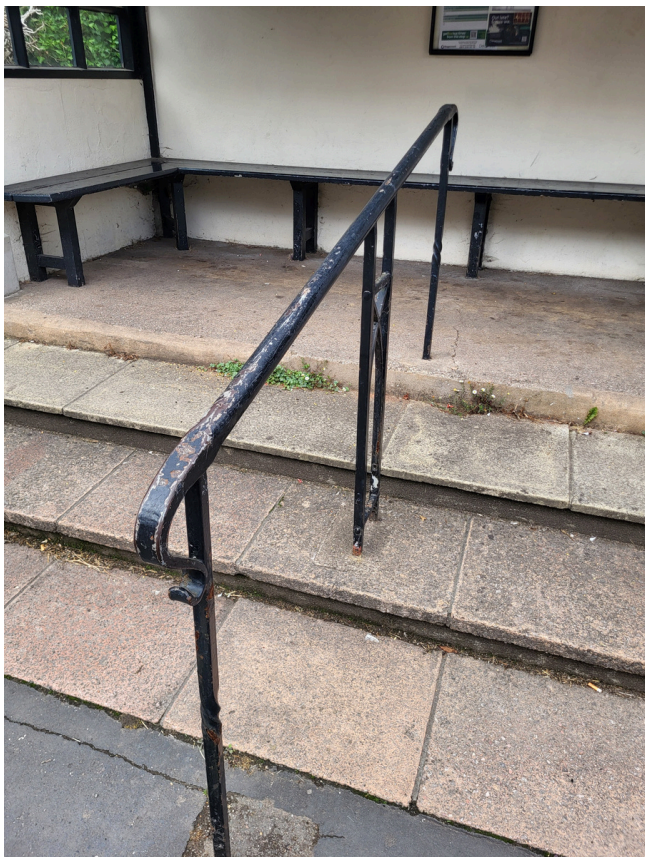
Image 3: Handrail requires coat of paint
