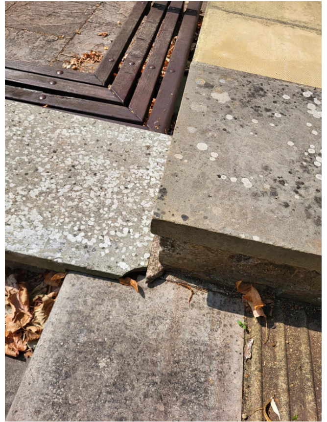
Image 10: Coping stone with broken corner
