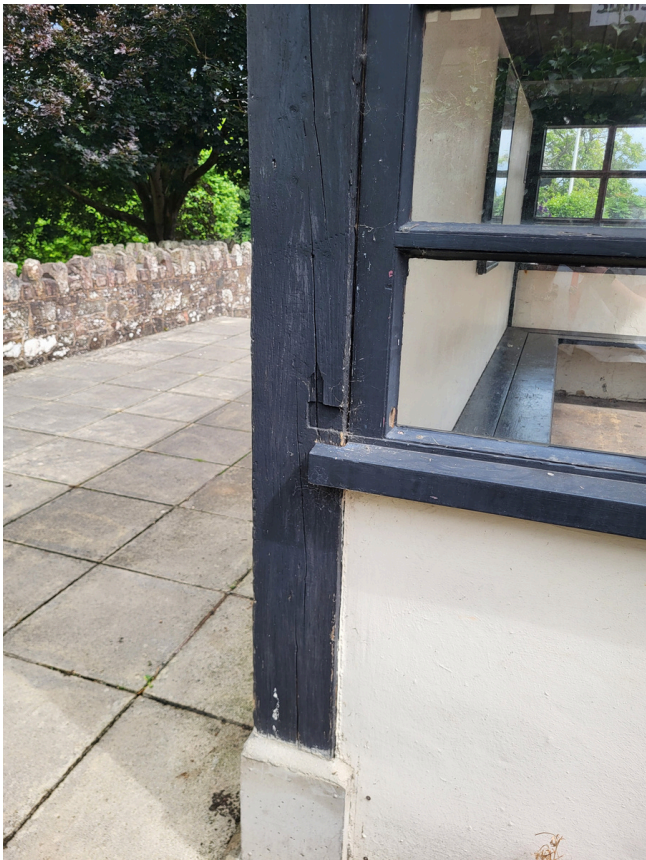
Image 9: No change in cracks to uprights
