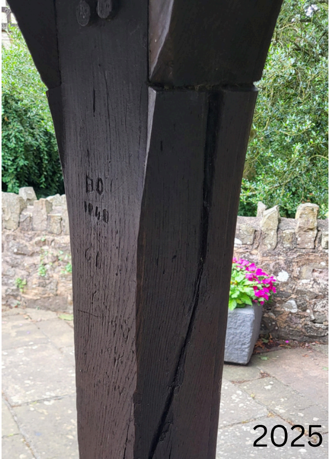
Image 7: Cracks to uprights. Comparison of 2024 and 2025.
