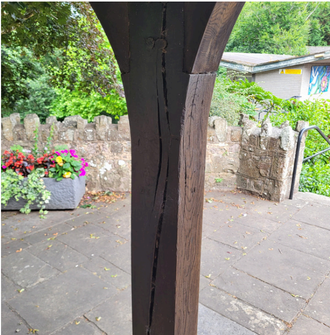
Image 6: Cracks to uprights. No change.
