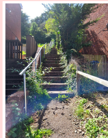
Newly installed handrail
