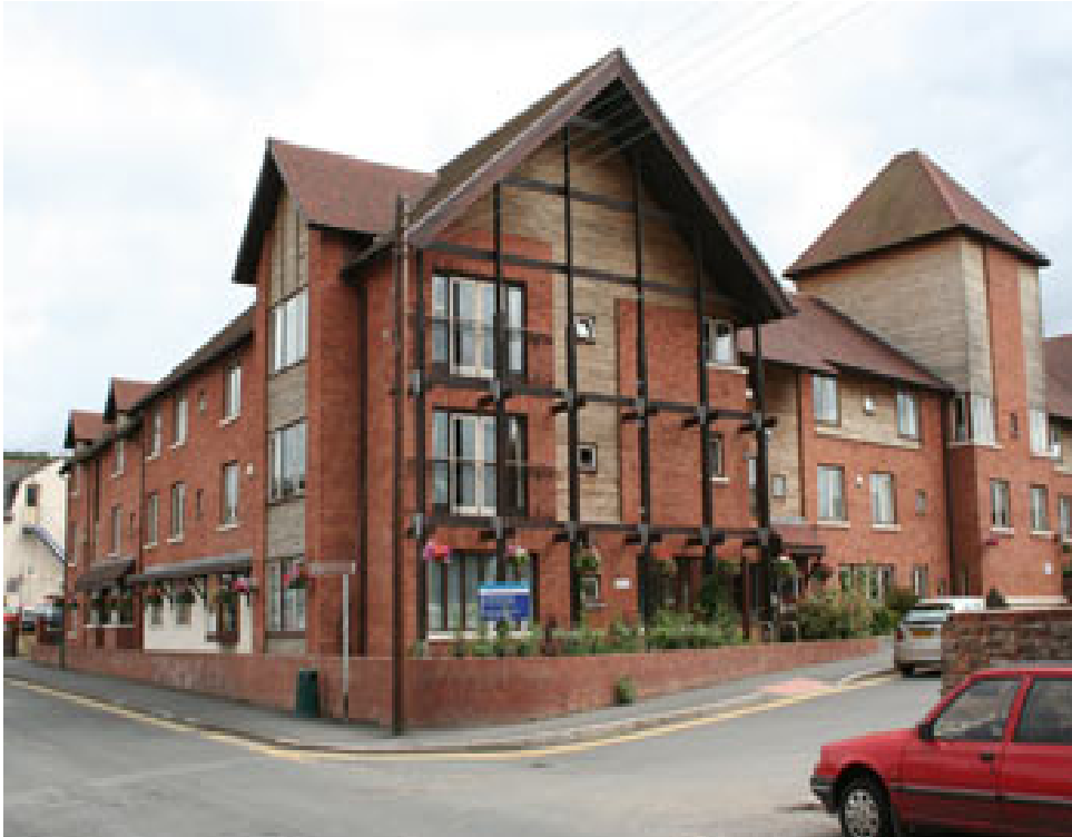
Ledbury Community Health and Care Centre
