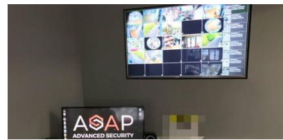
Control room equipment checking for general wear and tear including condition of user control panels and screens.
