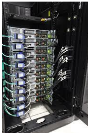
Server room hardware. Downloading system status logs to generate reports for the customer, applying system software updates.
