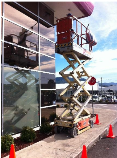
Field equipment using ASAPs safe, elevated working platform. Regular site safety talks with the client, ensures the highest safety levels.
